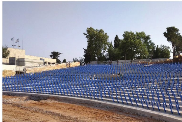
The site of the Park of Peace Amphitheater, Mevasset-Zion, Israel, was considered to have a moderately aggressive chemical environment due to direct exposure to the ground.
