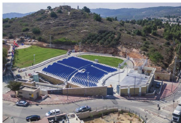
With a proximity of only 200 m (565 ft) from a main thoroughfare, there was a greater likelihood of early carbonation, which could reduce the naturally high alkaline environment of new concrete that initially protects rebar from corrosion at the Park of Peace Amphitheater site.
